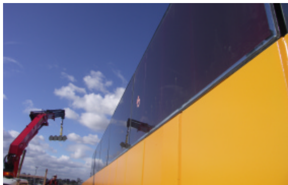
PV panels being installed above the concrete
