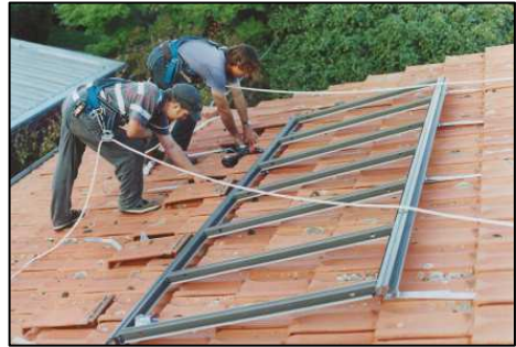
GS Contractors with safety harnesses
