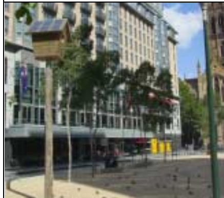
PV panels on the roof
