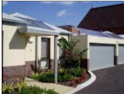
Solar Hot Water & PV Panels
