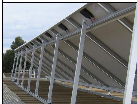
Framing Support Rails
