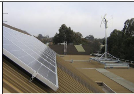
PV Panels & Wind Generator
